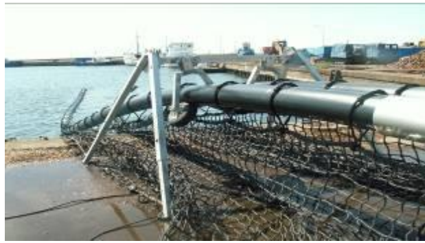
Figure 4. Top: The PVC pipes (in 12 m lengths) used for flotation is welded together inside a container. Middle: the net is stuck on automatically when the pipe is ejected and with Kalmar Castle in the background. Bottom: The farm unit is launched directly into the water.
